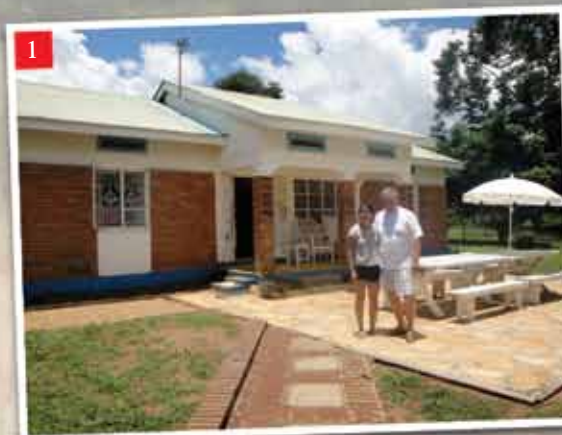
(1) Bery's Place. (2) The entrance to Korogwe Health Centre. (3) Wind-driven water pump in Korogwe. (4) Performing a hysterectomy - check out the size of the fibroid!
